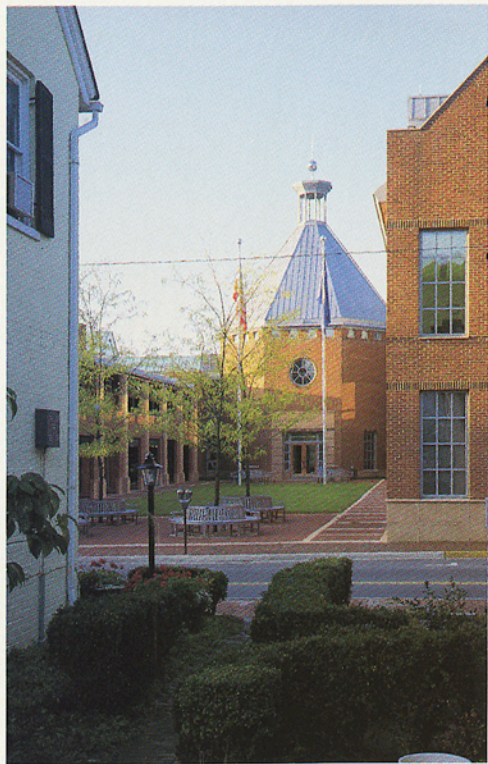
ABOVE: Architect Hanno Weber's plan for the government complex yielded many dividends, including a neatly defined urban plaza facing busy Market Street. BELOW: The center's three-story office building re-creates the urban edge along Wirt Street.
