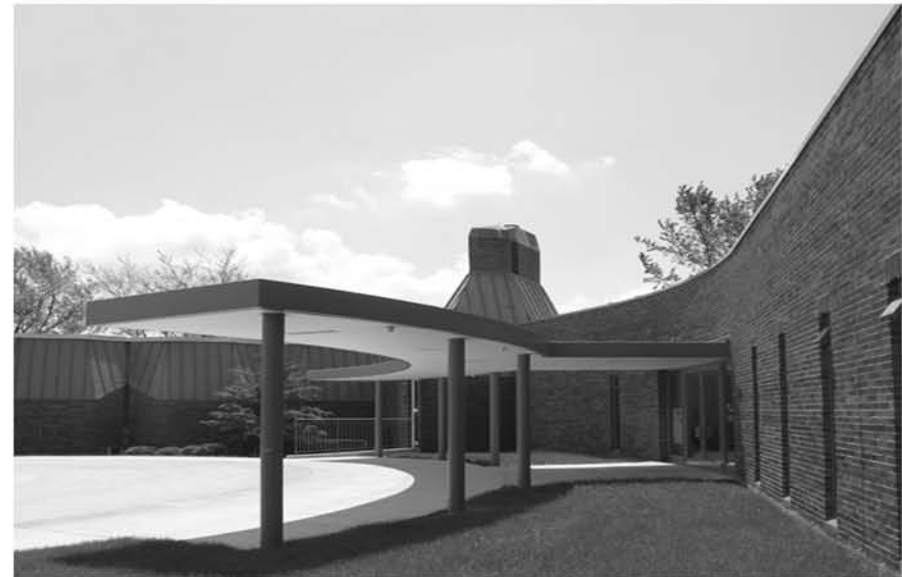
27. Completed Phase I Entrance Court Canopy
