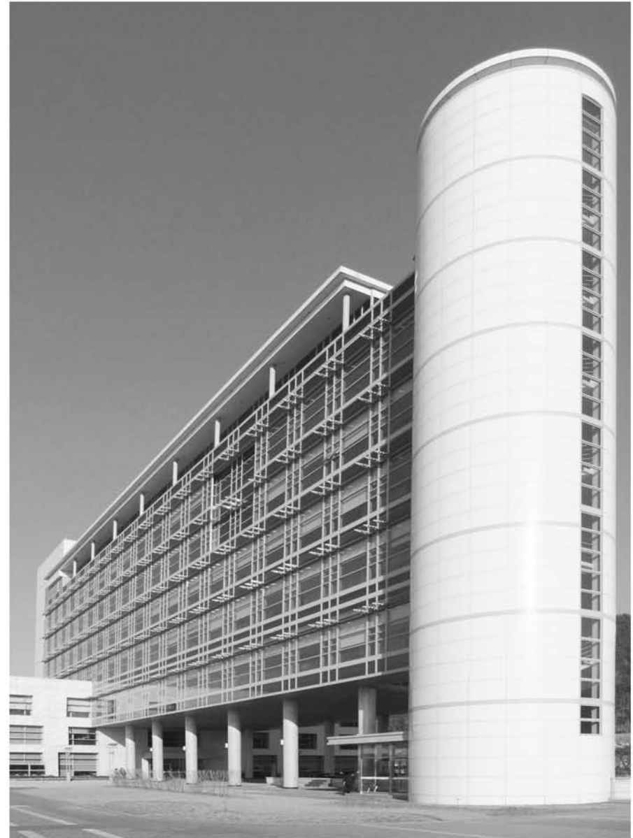
25. Administration Wing from the South
