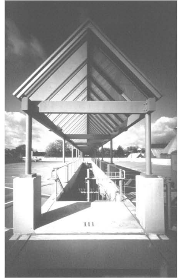
38. Parking Structure Skylights
