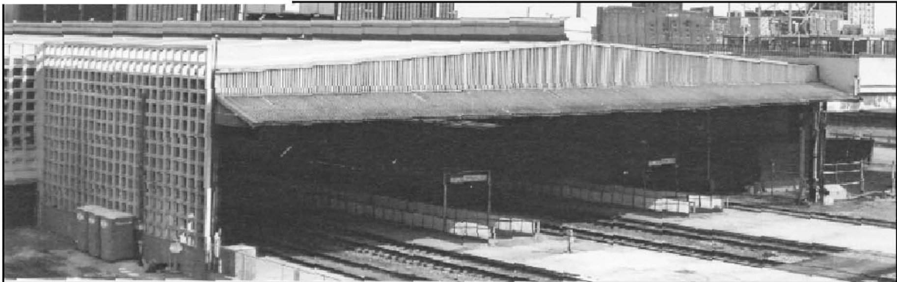
1. Existing Train Shed West Elevation
