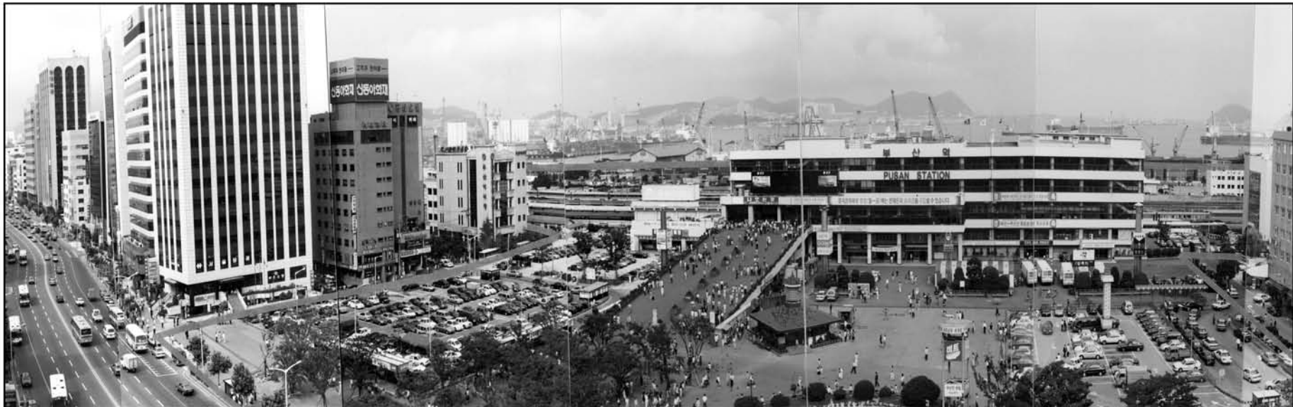
3. Existing Railroad Station & Plaza off Chung Ang Road
